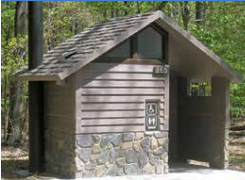
ROCKY MOUNTAIN Mocha Caramel Board & Batt Upper Walls Basalt Rock Lower Walls Mocha Caramel Cedar Shake Roof
