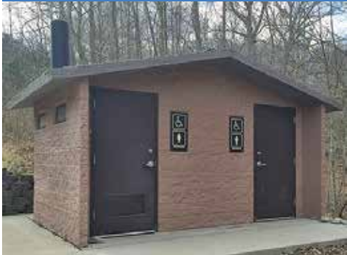
TIAGO SPECIAL Mocha Caramel Split Face Block Walls Malibu Taupe Cedar Shake Roof
